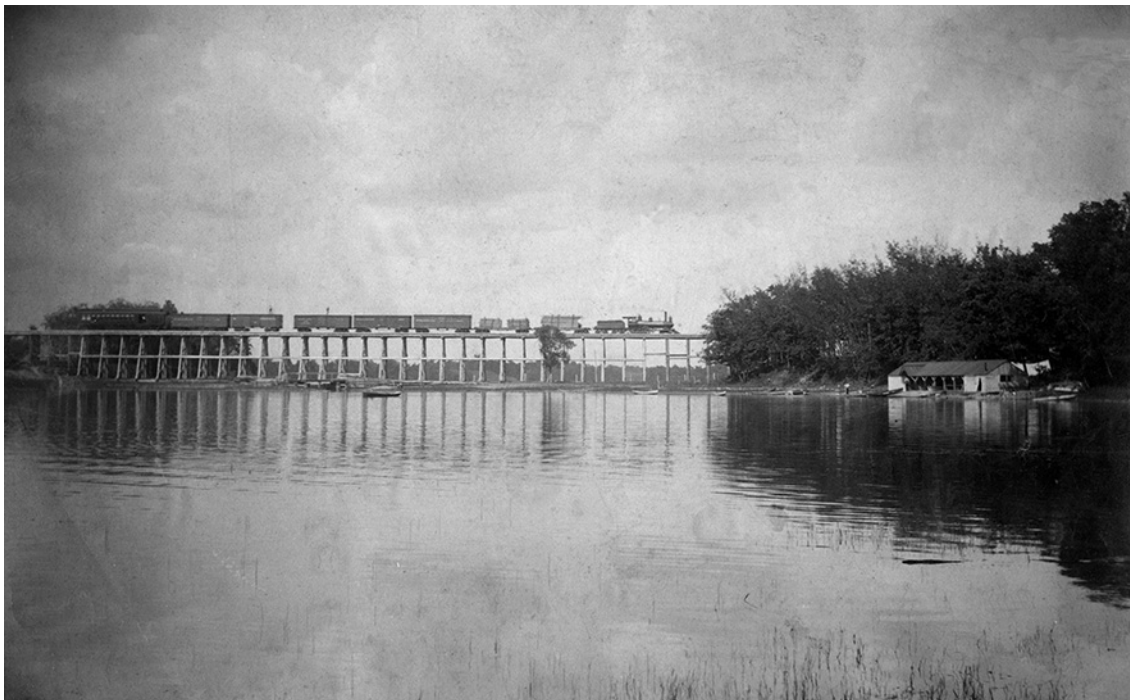
The new bridge with heavier construction. Imagine being a brakeman 40 feet above the ice in the winter in Minnesota!
