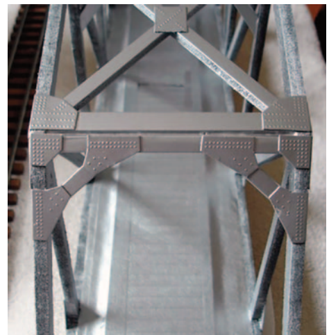
Painted end and top gusset plates with rivet details.
